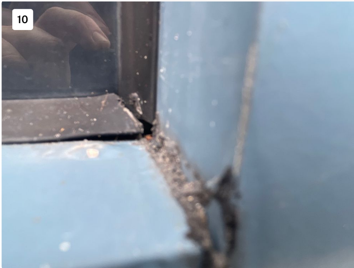
Openings at window seal corners
