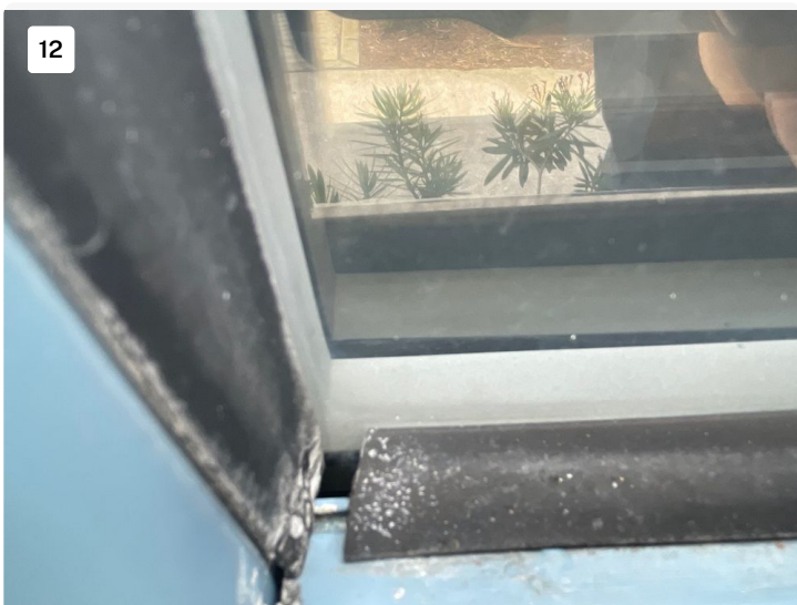
Openings at window seal corners
