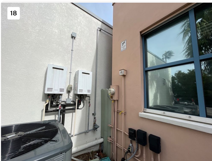
tight space between buildings on north side.
