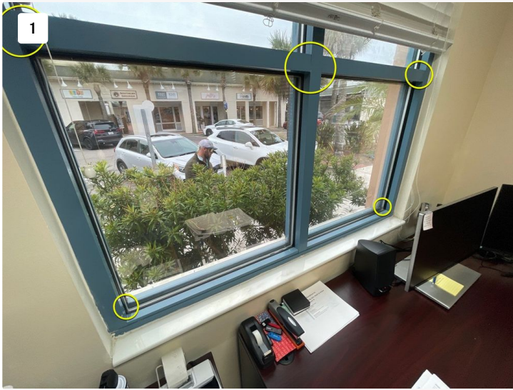
Water intrusion points illustrated
