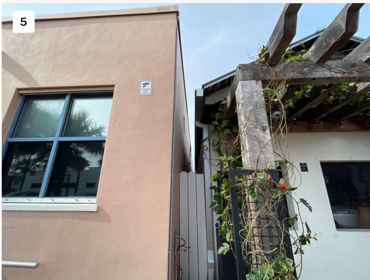
North side overview
