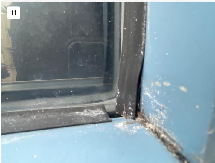
Openings at window seal corners
