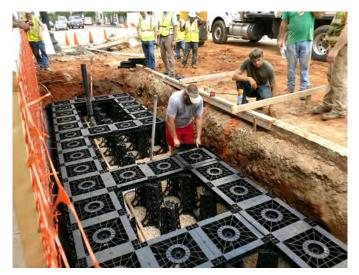
Figure 4.86: Tree wells with Soil Cells
