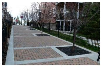
Figure 4.87: Pervious pavers with tree wells
