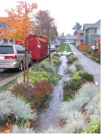
Figure 4.88: Bioswale filters stormwater
