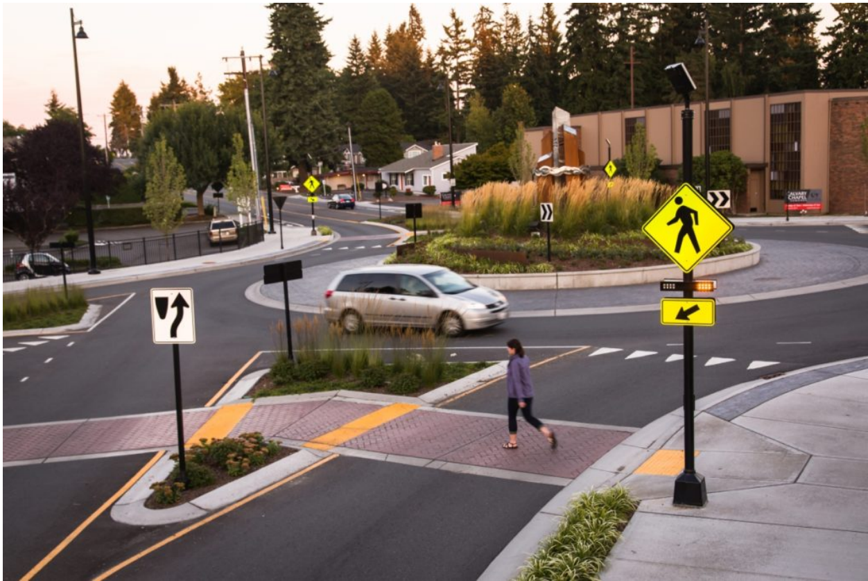
FIGURE 6 RRFBs at a single lane roundabout in Edmonds, Washington. Courtesy of Carmanah Traffic, https://carmanahtraffic.com/
