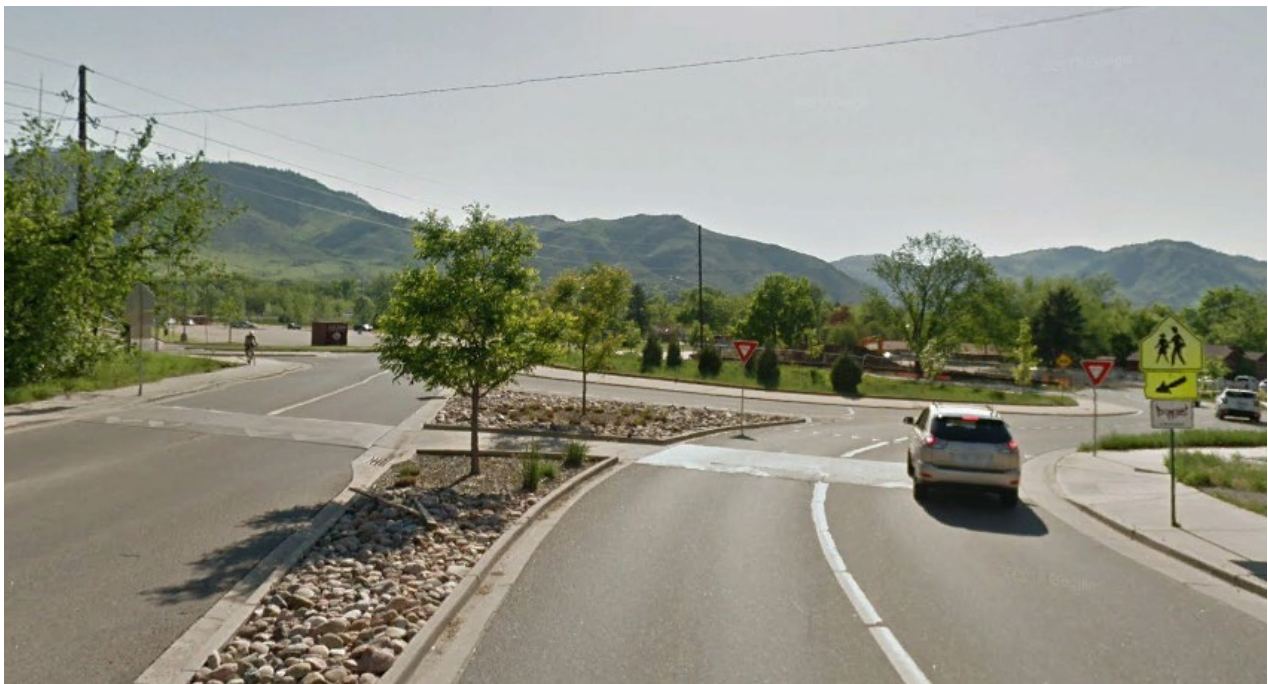
FIGURE 7 Raised crosswalk in approach to a roundabout in Golden, Colorado. From Google Maps.
