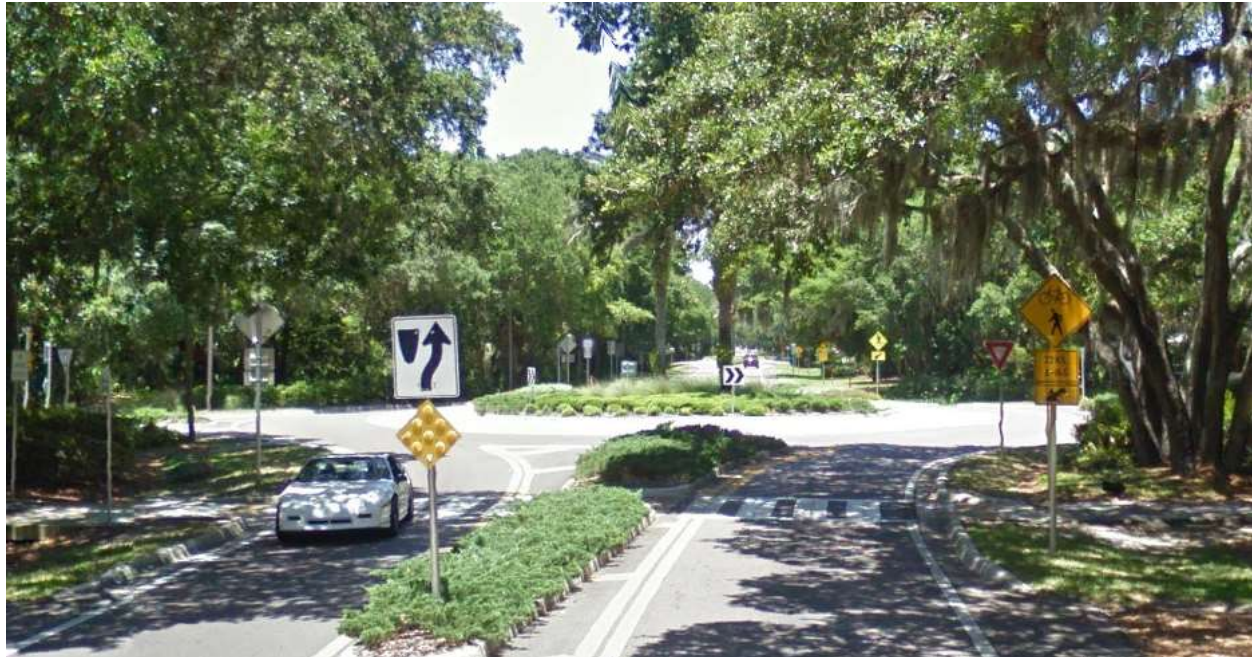
FIGURE 1 SR A1A at Beach Lagoon Road, Amelia Island, FL. From Google Maps.
