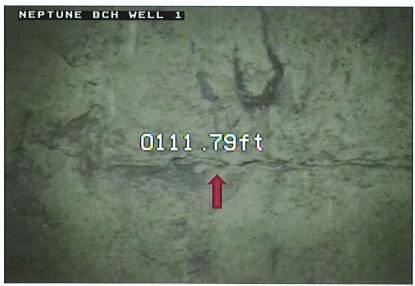
Photograph 2 - Typical Casing Joint at 111 feet
