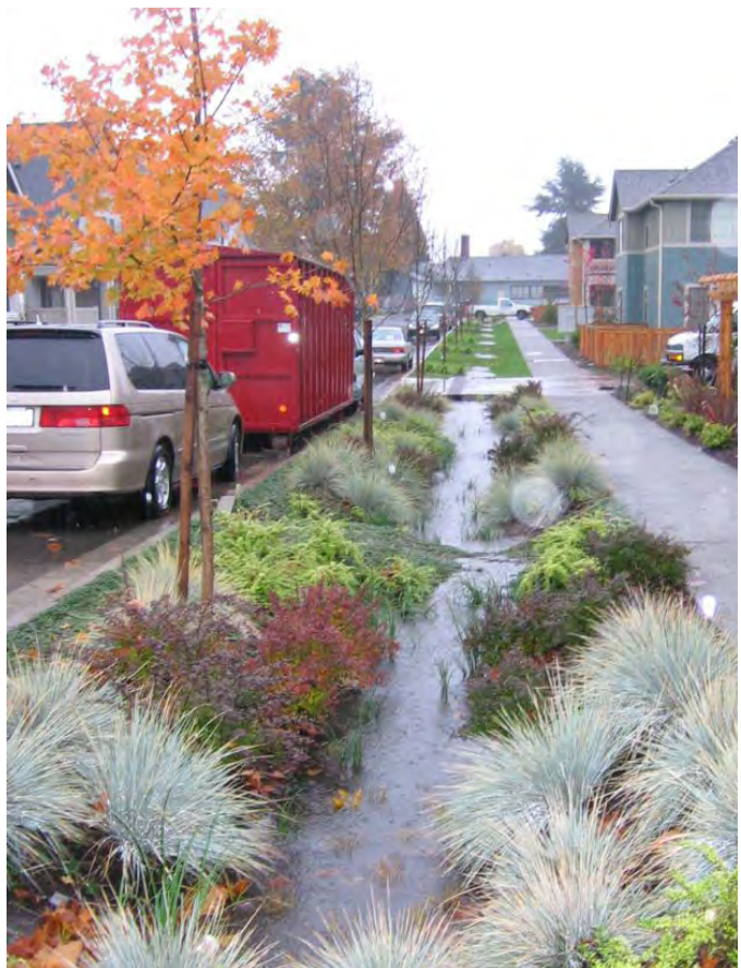
Figure 4.88: Bioswale filters stormwater
