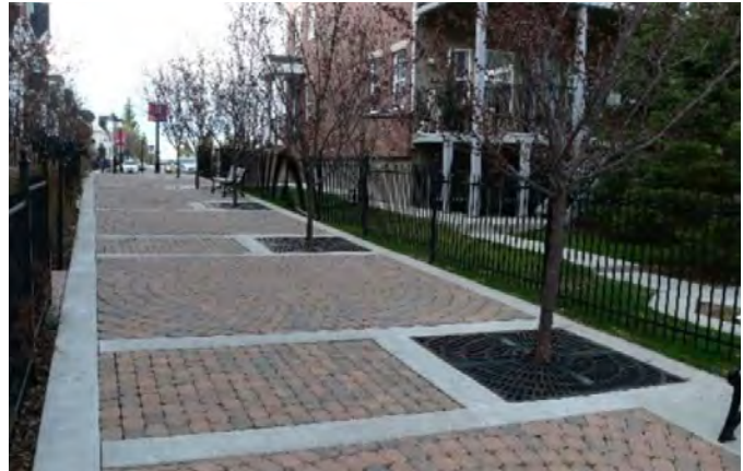
Figure 4.87: Pervious pavers with tree wells
