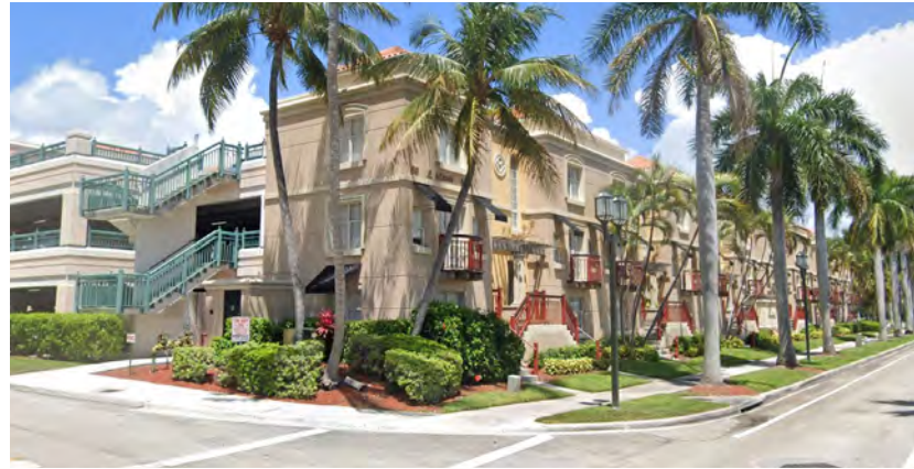
Mizner Park Townhomes Hide Parking Structure from the Street, Boca Raton, FL (Photo Credit: Google)
