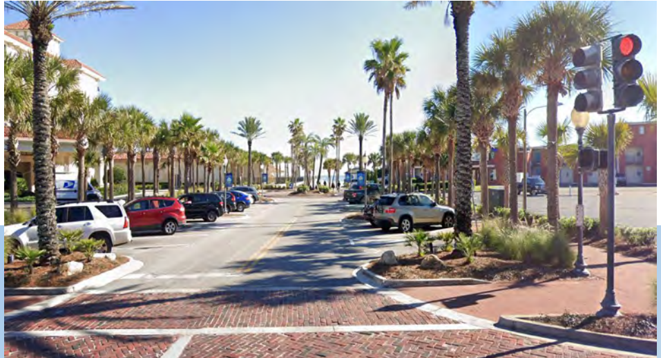
Figure 4.34: Atlantic Between 1st & Midway Street Existing Condition
