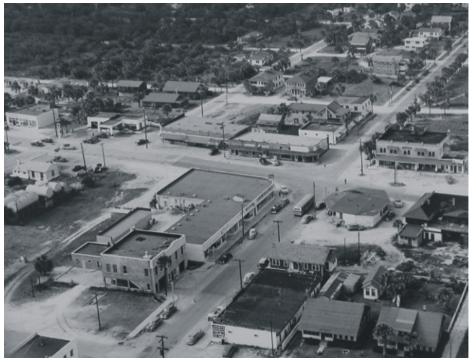
Commercial buildings on 1st Street and Atlantic, post WWII; Source: http://www.historicaltextarchive.com/sections_action_read_artid_447.html
