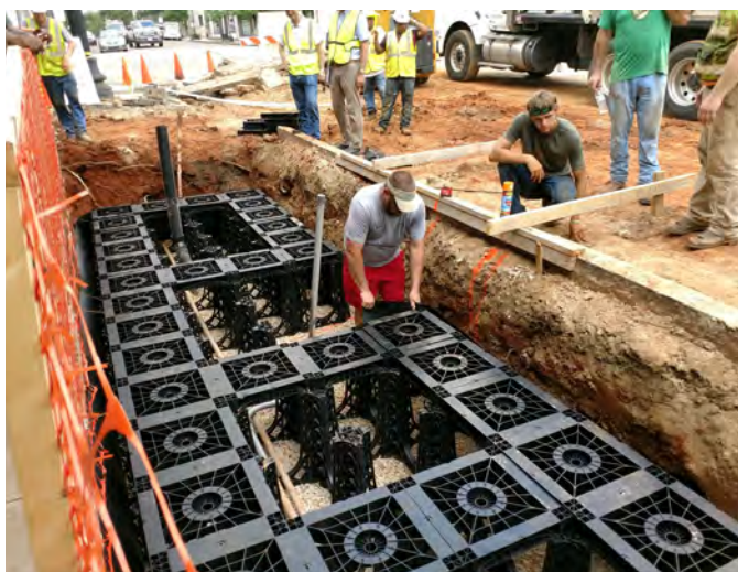
Figure 4.86: Tree wells with Soil Cells
