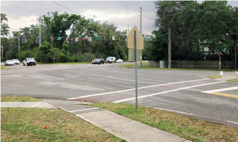
Figure 4.27: Penman & Florida Intersection: Existing Conditions
