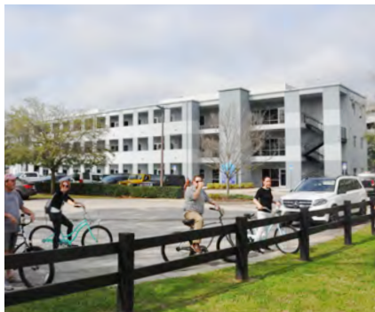
Sky Enterprises Office Building
