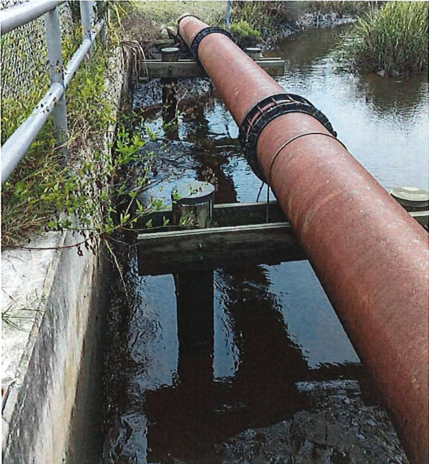
Combined Beaches 24" Effluent Force Main –Puckett Creek @ A1A (View to South)
